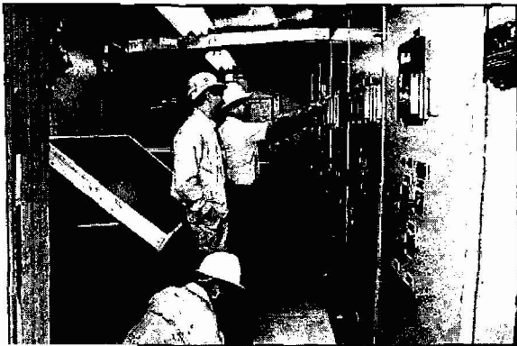
Syed Ahmed, David Elliott, and a UE customer service engineer inspect a substation control panel.
