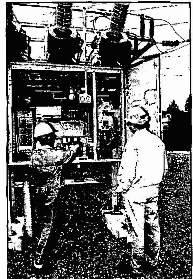
Syed Ahmed and David Elliott inspect a substation breaker panel.
