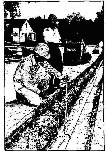
Gas Safety Staff members John Kottwitz and Amy Brox check for compliance during natural gas pipeline installation.
